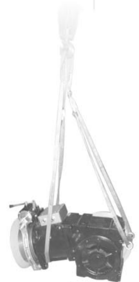
5. LIFT TRACTION MACHINE & PUT IN MACHINE ROOM
